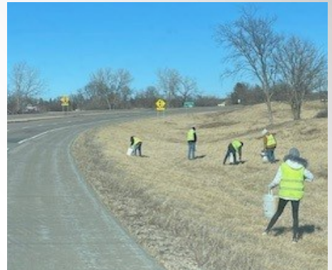
HWY 61 Ditch Cleaning
